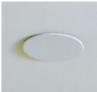
Breakthroughs in technology have allowed fire sprinklers to be more affordable and easier to install in homes than ever before. With a variety of designs available, sprinklers blend into the interior decor with ease. And, fire sprinklers usually operate off the domestic water supply.
